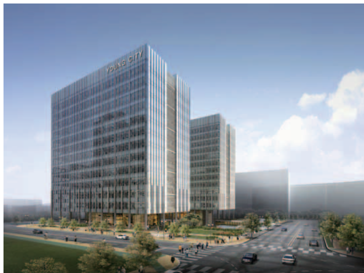
Mullae Office Building (Korea)
