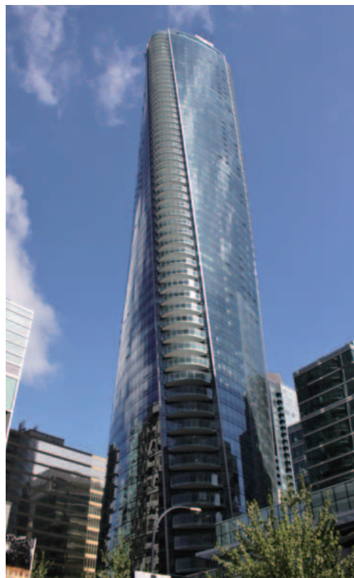
Trump Tower International Hotel & Tower® Vancouver (Canada)
